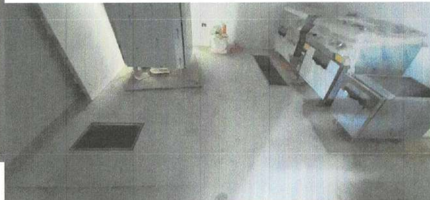
INSTALLATION OF FLOOR DRAIN – DIETARY AREA
