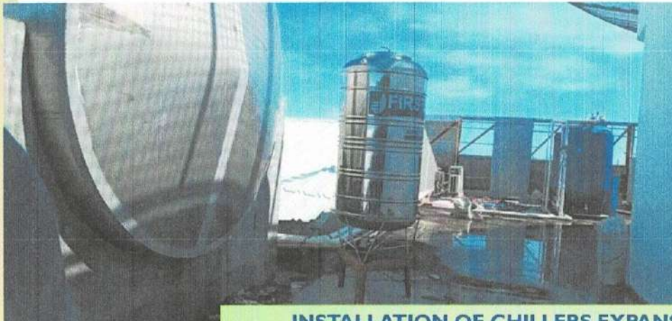
INSTALLATION OF CHILLERS EXPANSION TANK
