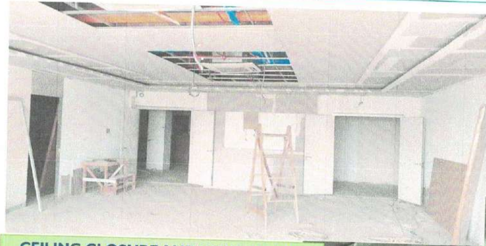
CEILING CLOSURE AND WALL PANELS
