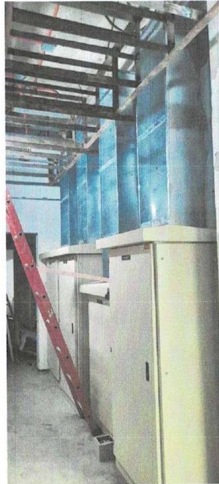
CHILLER PANEL POSITIONING & TRUNKING
