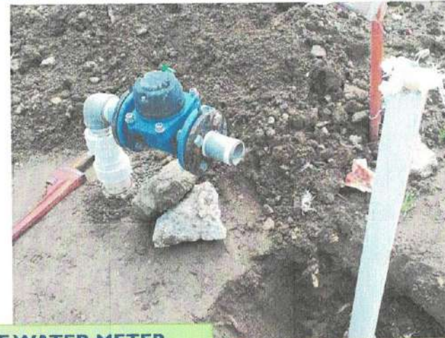
FINAL CONNECTION OF WATER METER
