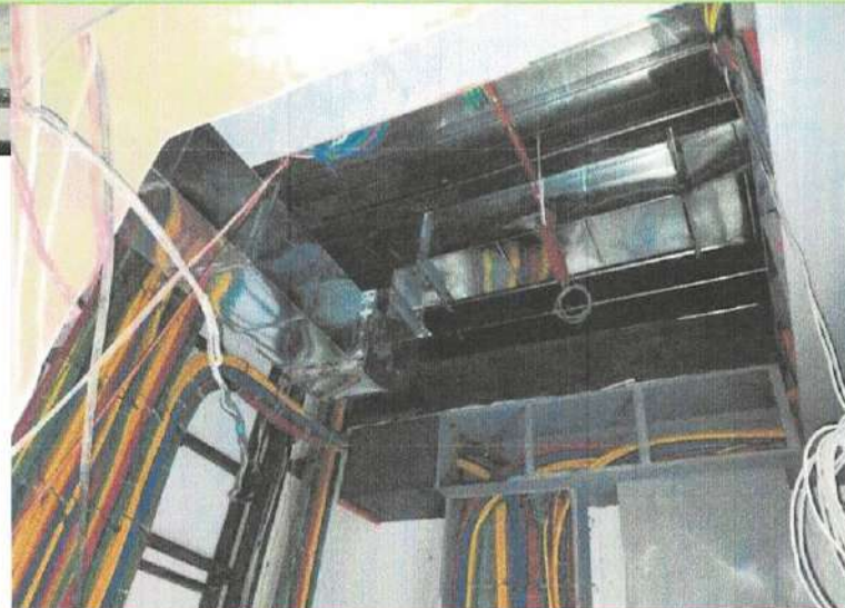
RETURN AND EXHAUST AIR DUCTING AT 6F ISOLATION ROOM
