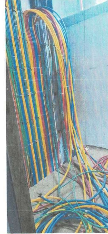
INSTALLATION OF FEEDER LINES FROM POWER HOUSE TO 4 TH FLOOR
