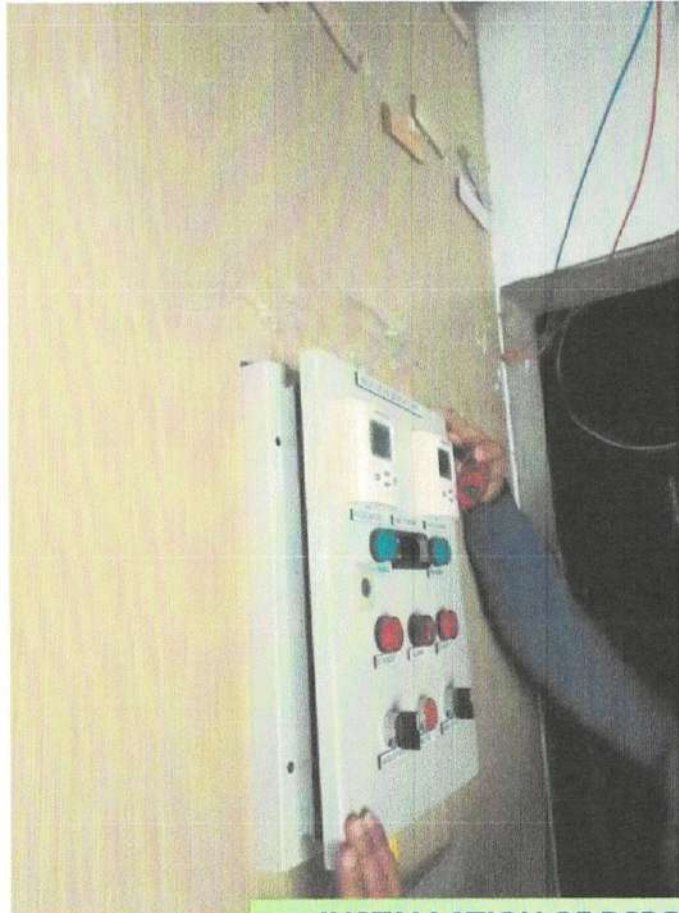
INSTALLATION OF DSPC CONTROLLER – ISOLATION ROOM
