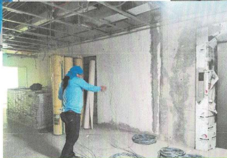
INSTALLATION OF LIGHTING
