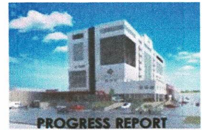
PROGRESS REPORT As of May 30, 2023
