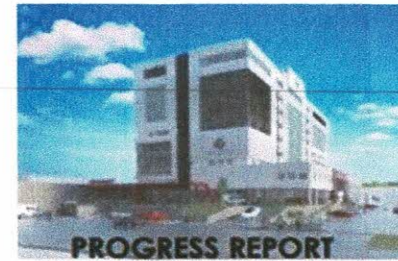
PROGRESS REPORT As of May 30, 2023
