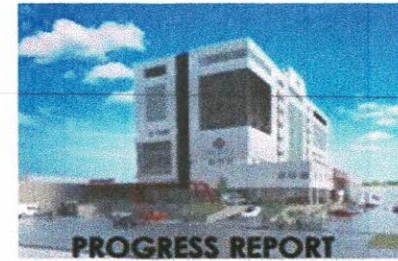
PROGRESS REPORT As of May 30, 2023
