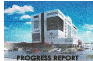
PROGRESS REPORT As of May 30, 2023
