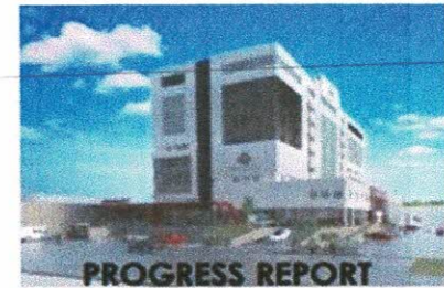
PROGRESS REPORT As of May 30, 2023
